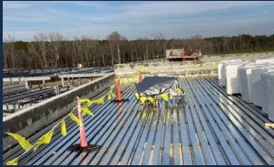
Roof material staging for install at gym high roof
