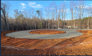
Stone placement for driveways and roundabout
