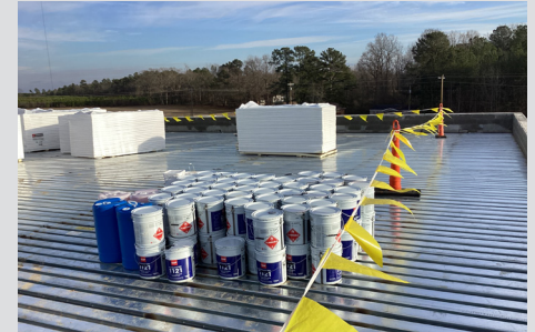
Materials are staged before installation. The cans above are a Bonding Adhesive, which is placed between the fasteners and the TPO membrane.
