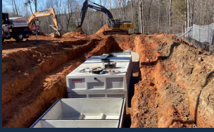
Septic tank installation
