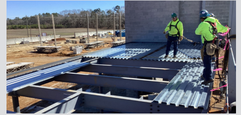
Roof decking must be installed before the TPO roof system.
