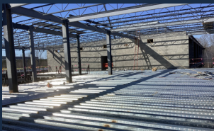
2nd floor decking ongoing (Area A)
