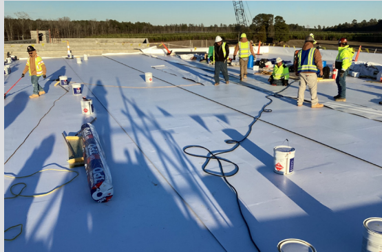
TPO roof membrane installation at Area D - gym
